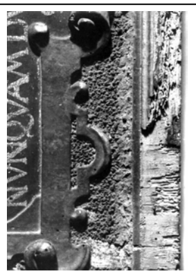
Fig. 5. Anobium punctatum attack on wood pieces.
