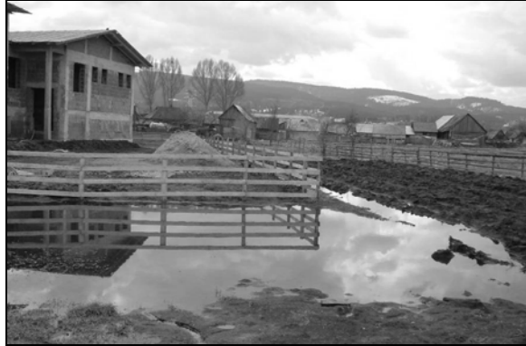
e. The surroundings of the building are flooded; note the filled area in the fenced corner. (3.04.2006)
