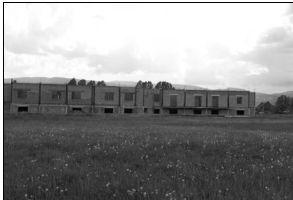
d. Constructions on pond C were halted by lack of funds. (27.05.2005)
