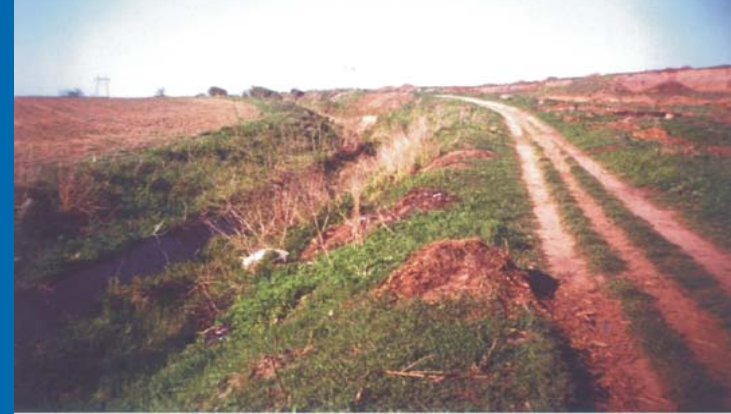
Abandoned irrigation channel, Sadova (May, 2002)
