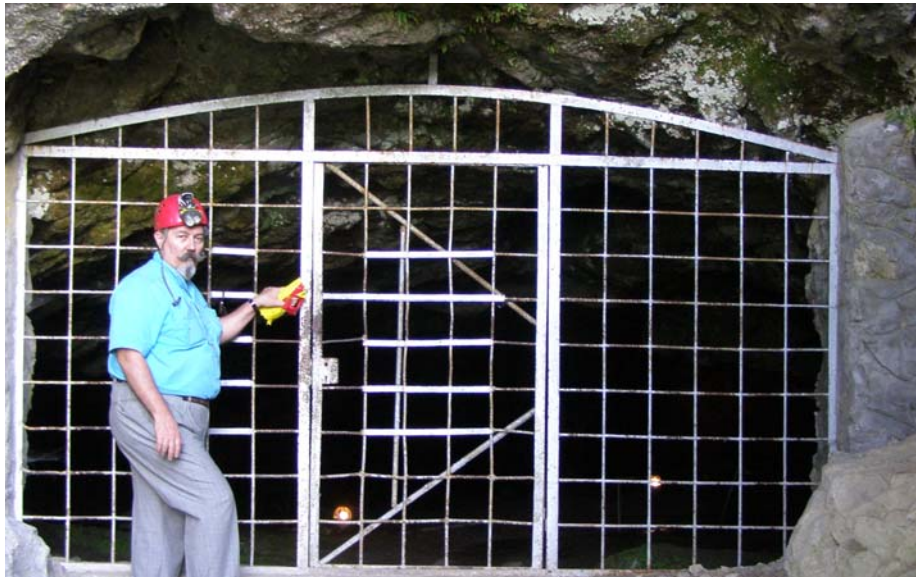
Fig. 11. Southern entrance with an actually unsuitable gate (15 × 15 cm net of lattice) not allowing bat flying access.
